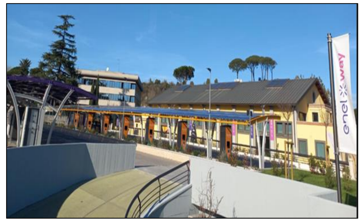
7 - XLAB Photovoltaic shelter in EV parking
