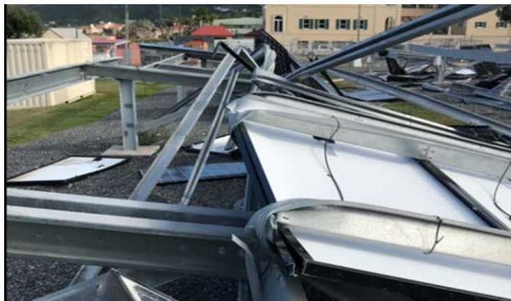
Figure 10. It might be the responsibility of the O&M provider to respond and ensure that storm damage is rendered safe both in terms of electrical hazards and loose components following an extreme weather event such as this damage in St. Croix in 2017. Photo by Andy Walker, NREL
