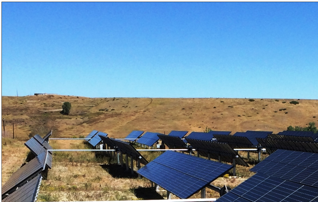
Figure 5. Although improving annual energy delivery, especially in summer, tracking mechanisms and controls require regular maintenance to be effective (photo by Andy Walker).
