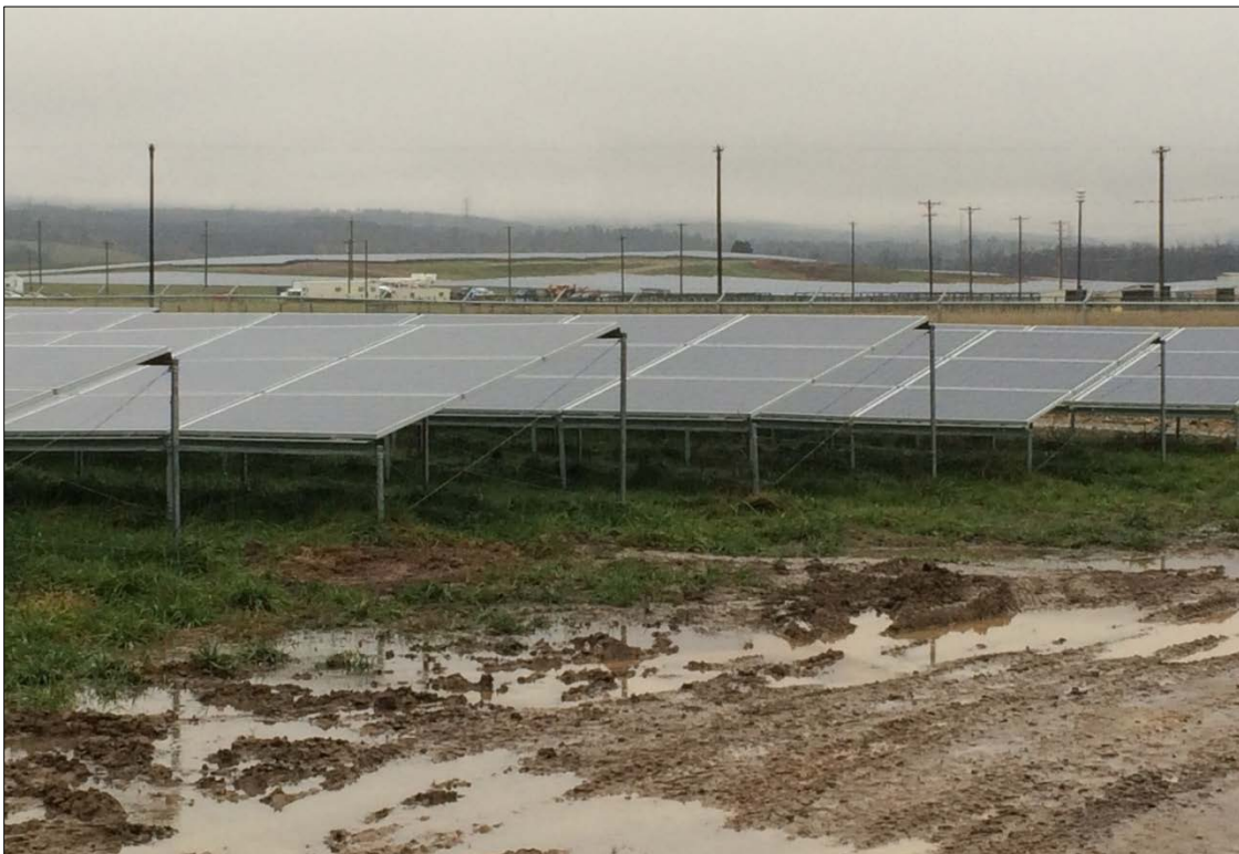
Figure 4. Drainage and storm-water run-off are difficult to improve after the PV array is installed, requiring diligence in design and construction of storm-water management systems (photo by Andy Walker)
