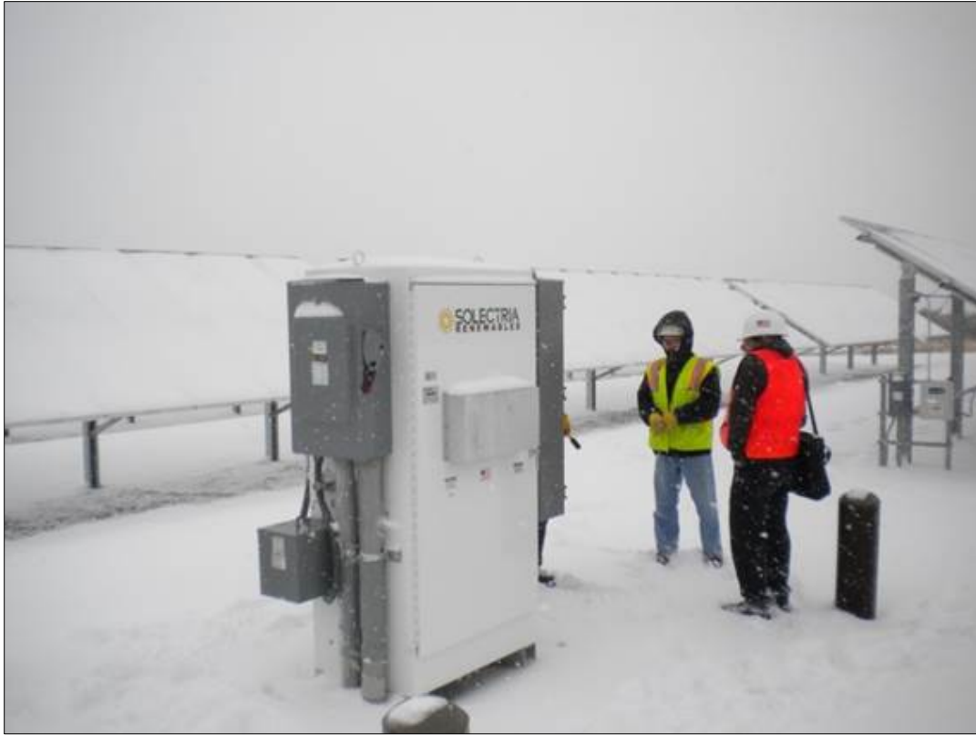
Figure 8. Snow is an environmental condition that both reduces performance and complicates provision of O&M services. (photo by Andy Walker)
