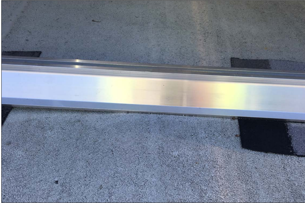
Figure 2. Best practice is to run slip sheet continuously under rack members to avoid direct contact with roof membrane. In this photo, direct contact of the rack is cutting into the roof surface (photo by Norm Crouse, courtesy of Lightbox Energy)
