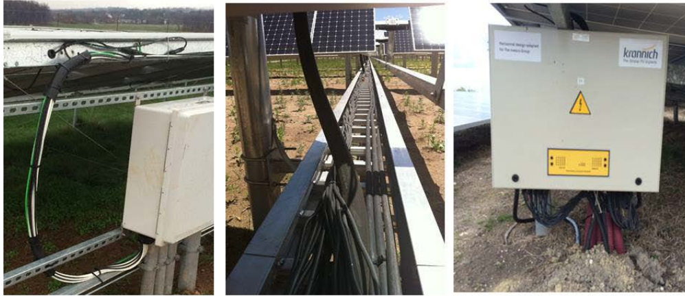
Figure 1. Maintenance of wire management systems depend on plastic wire-ties and grommets which can break or pinch wires (left), exposure to sunlight, wind and weight of ice (center), and access by chewing rodents (right). (photos by Andy Walker)
