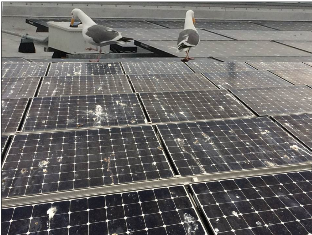
Figure 7. Bird populations are a source of soiling, as well as nests that need to be removed, and seeds that can sprout on arrays. (photo by Andy Walker)
